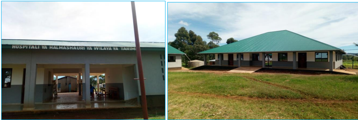
Picture 29: Hospital building in Tarime District, sponsored by Acacia's North Mara Gold Mine
