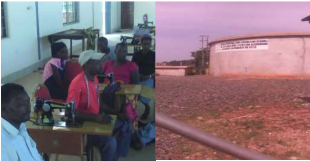
Picture 24: Some of the projects funded by GGM
